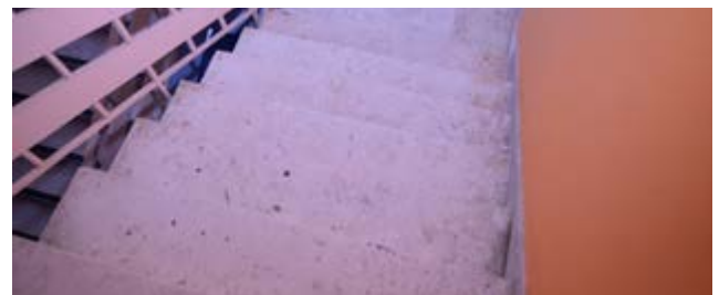
Figure 1.5 Contrasting edge strips on stairs enable PVIs to better judge position and height of steps. Photos: Ameen Harb.
