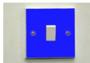
Figure 1.6 Contrasting light switches and sockets can be easier to find. Photos: Ameen Harb.
